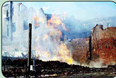
Building burns as result of gas explosion.
