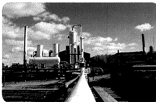
EOR operations in Michigan. (Courtesy of MRCSP)
