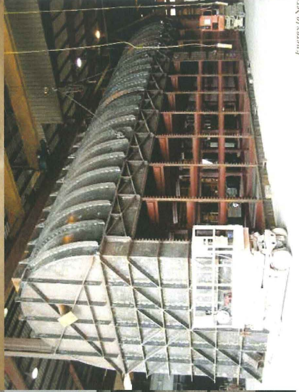
Dryer Housing Cover 09/15/2011 09:45
