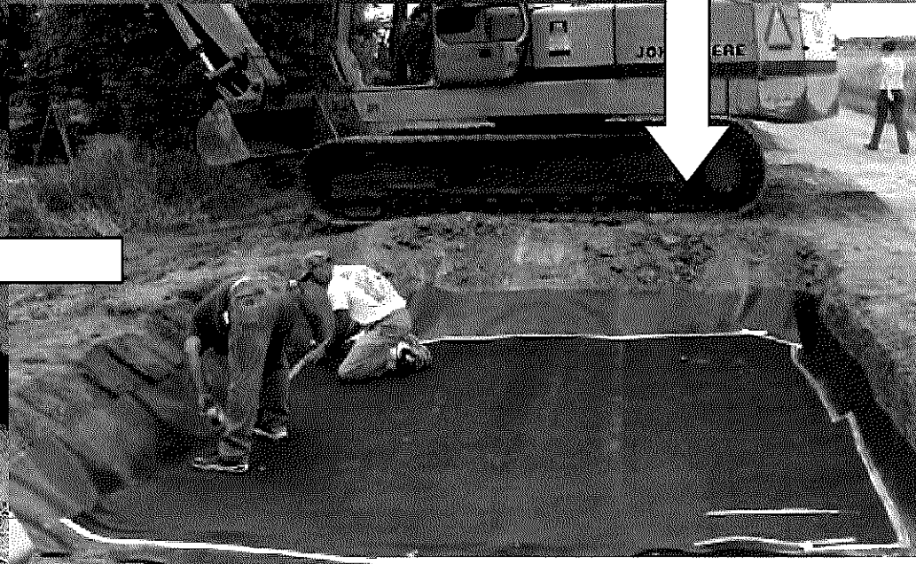
Drainage layer installation
