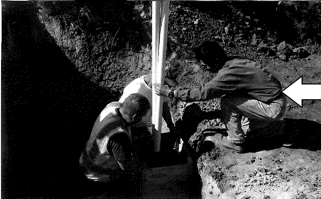
Collection tank installation
