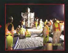
By 1:00 a.m., the pavement had been removed so the site could be prepared. Workers installed a polyethylene vapor barrier to mitigate water intrusion from the substrate as well as act as a bond breaker between the adjoining slabs.
