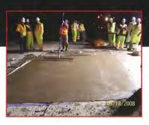
A grooving tool was applied to the surface of the **GreatWhite**<sup>TM</sup> material as it reached initial set. This step was completed at 2:00 a.m., - 40 minutes after placement of **GreatWhite**<sup>TM</sup>
