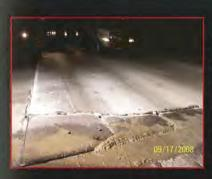
This deteriorated section of U.S. Highway 101 in Gilroy, CA. was selected to be replaced using concrete made with **GreatWhite™ Rapid Cement**. Traffic was diverted to the adjacent lane starting at 8:00 p.m., so that the 12 x 15 ft. section of 9 to 11 in. thick concrete pavement could be sawcut into manageable sections.
