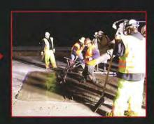
At 1:25 a.m., a vibrating screed was used to quickly strike off and level the concrete.
