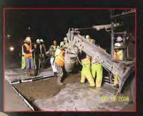
Placement of **GreatWhite™** began at 1:20 a.m. The mixer was calibrated off site prior to the placement.
