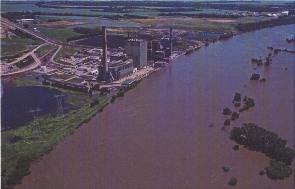
Power plant in floodwater:
