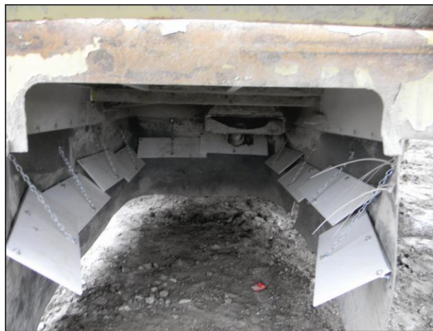
Figure 3.12. Air-blocking shelf with modifications incorporated into installation. This shelf was installed in short sections in an attempt to prevent potential damage that could occur during tramming with the drill mast up. Note that each of the sections overlap, eliminating any gaps in the shelf perimeter.
