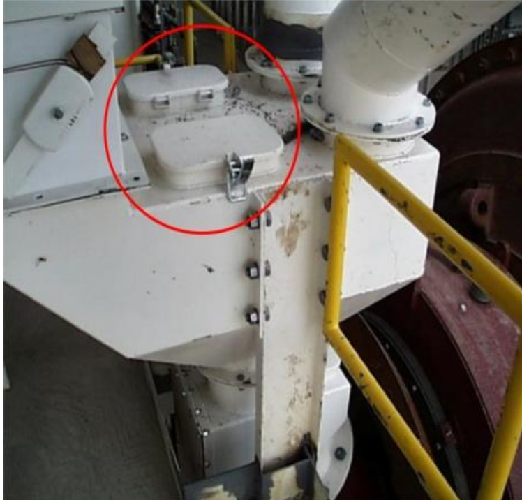
Figure 4.14. Sampling doors located on top of a collection/transfer point to prevent leakage.
