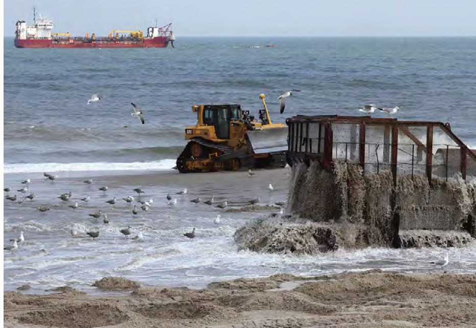
Discharge pipe with screen, construction equipment, and hopper dredge. © BOEM
