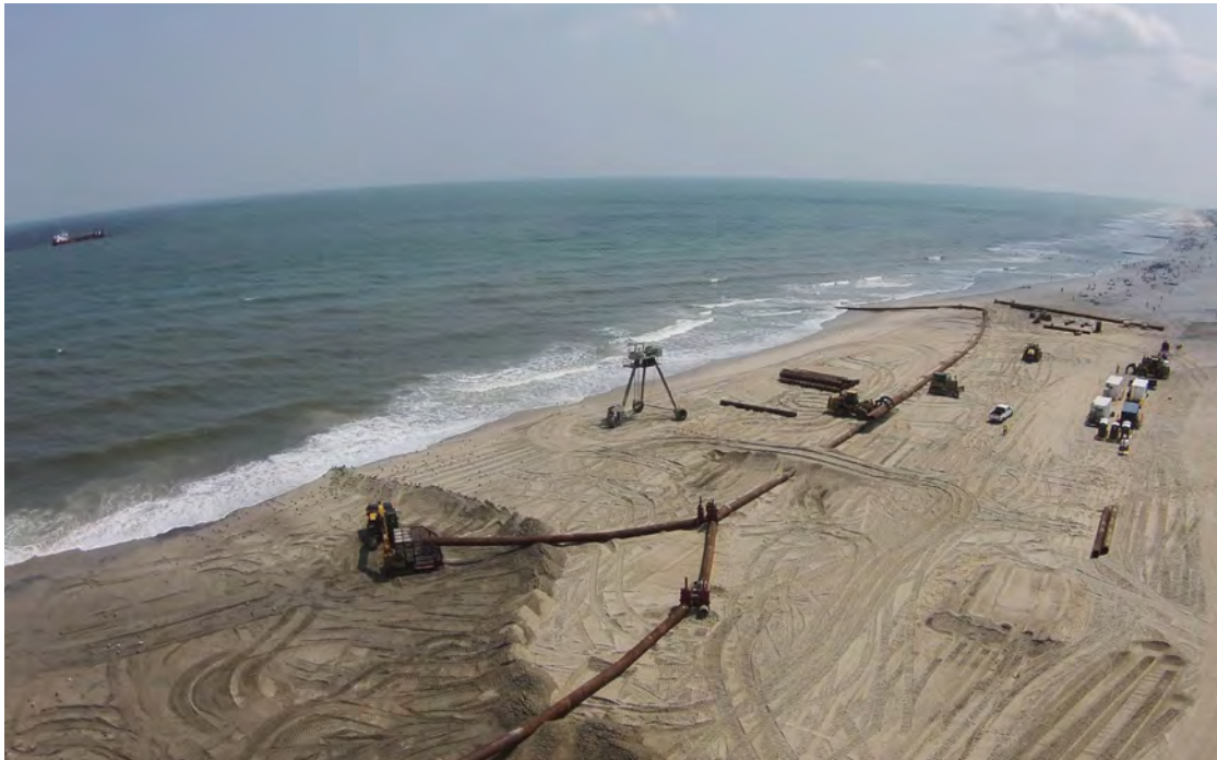
Aerial photograph of a beach nourishment project on Long Beach Island, New Jersey. © BOEM
