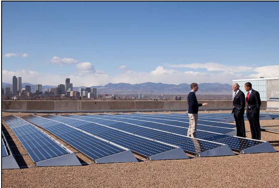
President Obama and VP Biden with rooftop PV arrays, Denver
